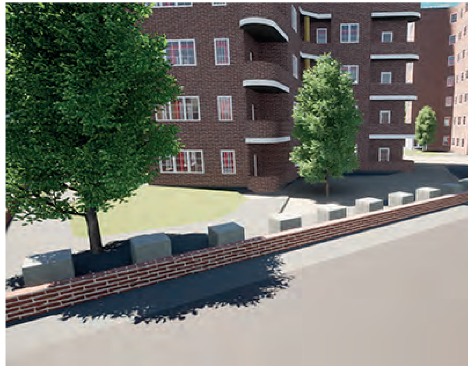
1. Kentledge blocks are installed
