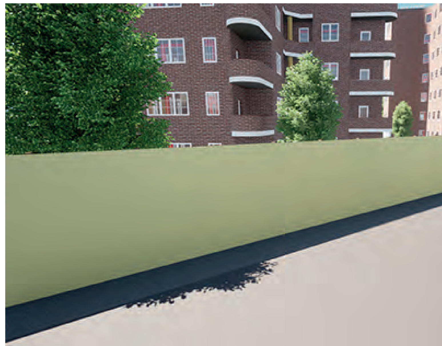
3. 3m high plywood is then attached
