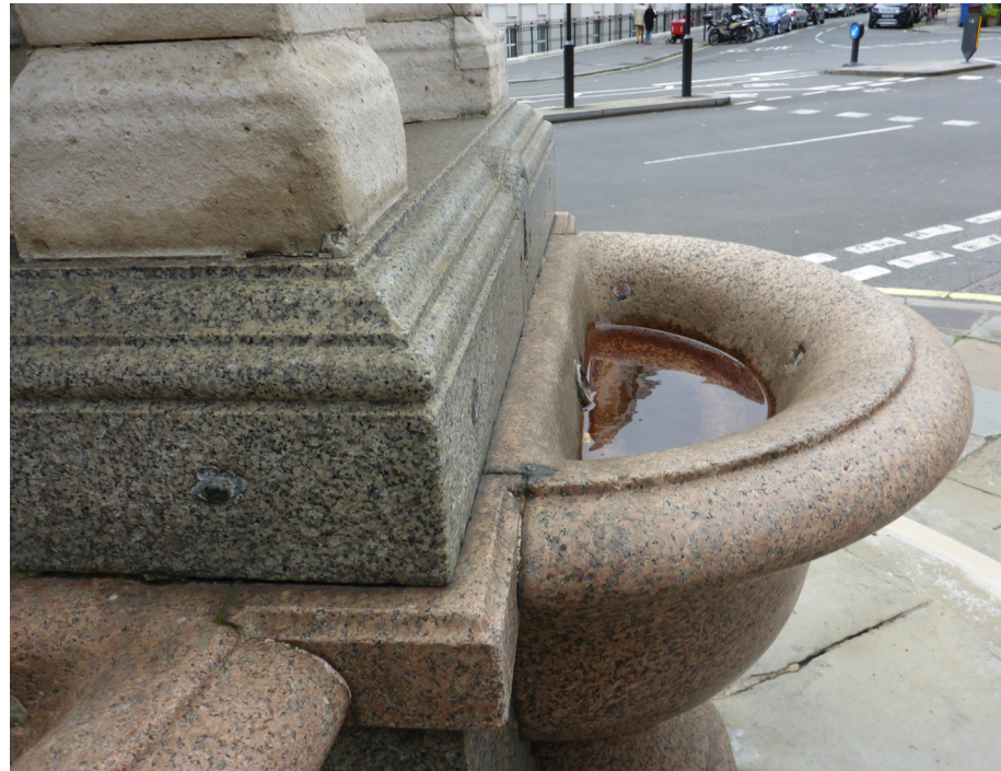
Fountain plumbing does not function properly
