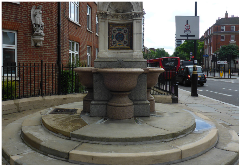
Yorkstone base of fountain suffers from poor drainage and shoddy repairs
