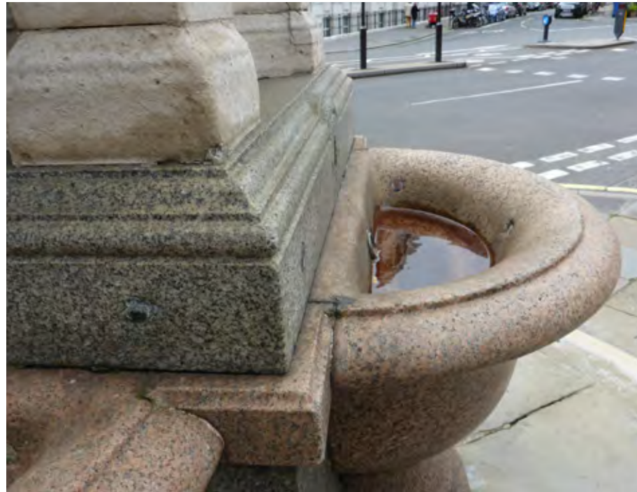
Fountain plumbing does not function properly
